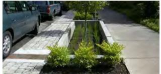
Image: Porous pavement and rain garden to filter stormwater. (Source: Pinterest)
